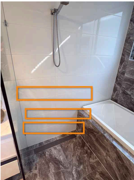
1st Floor Bathroom
