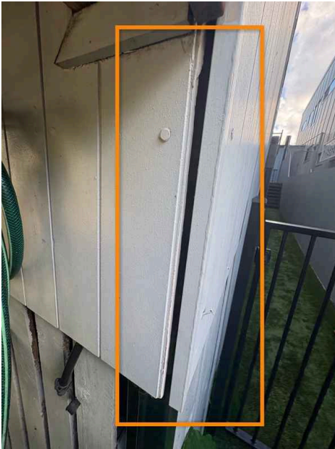
Ground Floor Rear
